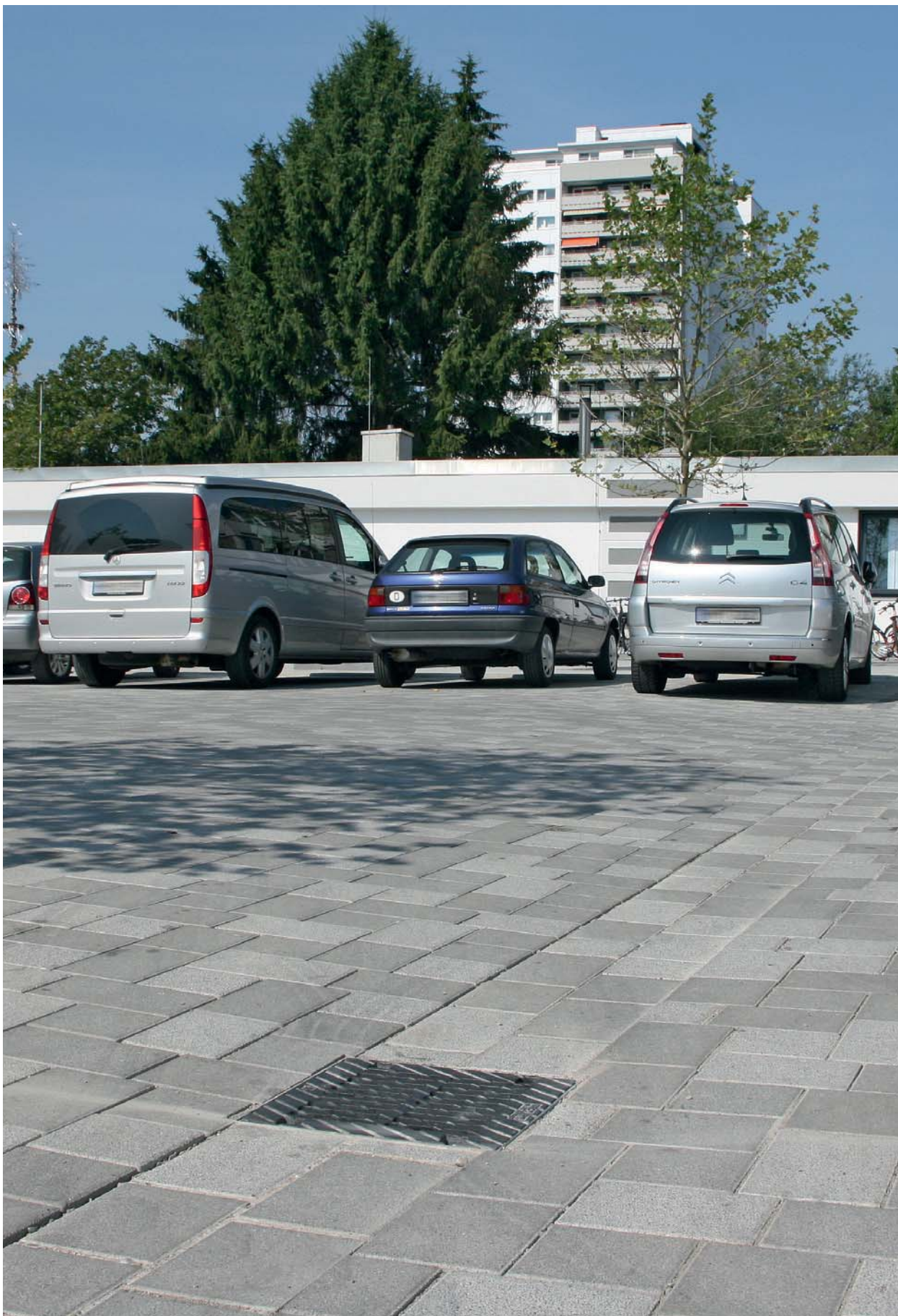
Reliable BIRCOsir point drainage at Machnigplatz in Memmingen.
