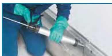
5. Applying the joint sealant
