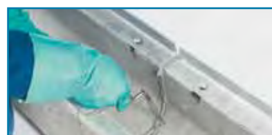
6. Smoothing the surface of the sealed joint
