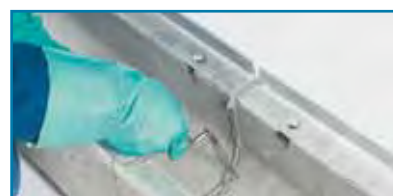
6. Smoothing the surface of the sealed joint
