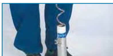
4. Mixing the joint sealant
