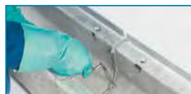
6. Smoothing the surface of the sealed joint
