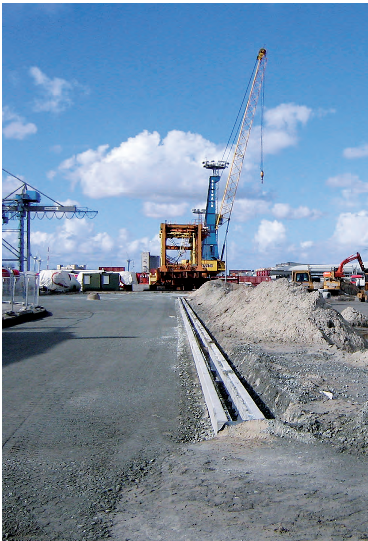
BIRCOsolid box channel during construction work at the Emden Northern Quay
