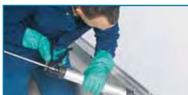
5. Applying the joint sealant
