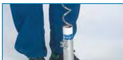
4. Mixing the joint sealant
