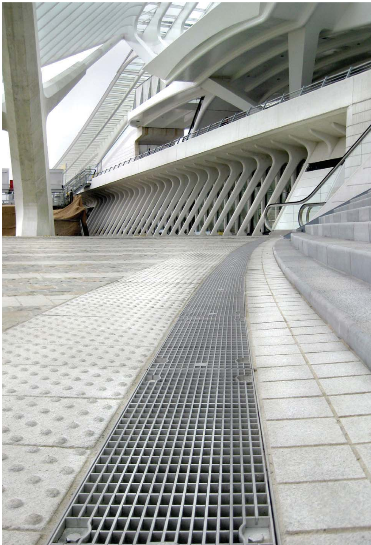
BIRCOprofil surface drainage at the high speed train terminal Luettich/Belgium
