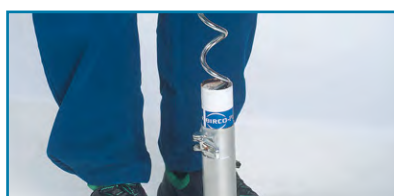
4. Mixing the joint sealant
