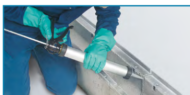
5. Applying the joint sealant
