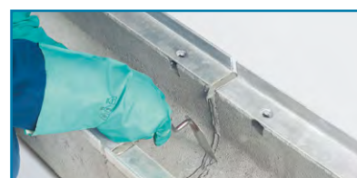
6. Smoothing the surface of the sealed joint
