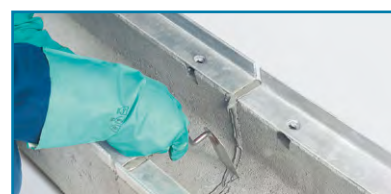
6. Smoothing the surface of the sealed joint
