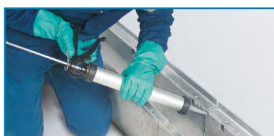
5. Applying the joint sealant
