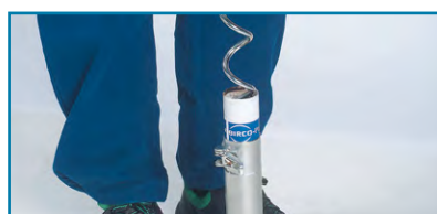
4. Mixing the joint sealant
